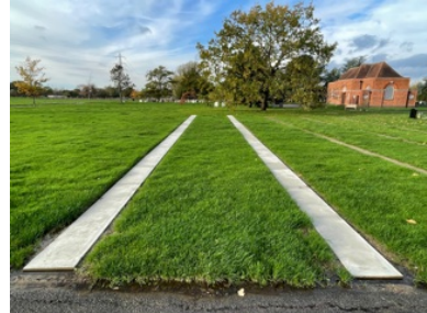
NEW MEMORIAL LANDING BEAMS
